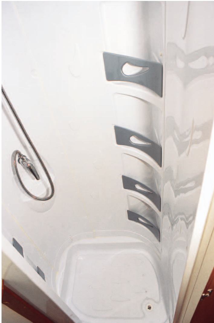
No riser for the showerhead, only a swivelling bracket in the otherwise excellent separate shower.
